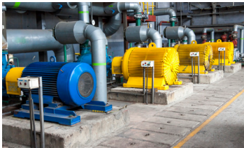
Plant / Equipment Installation
